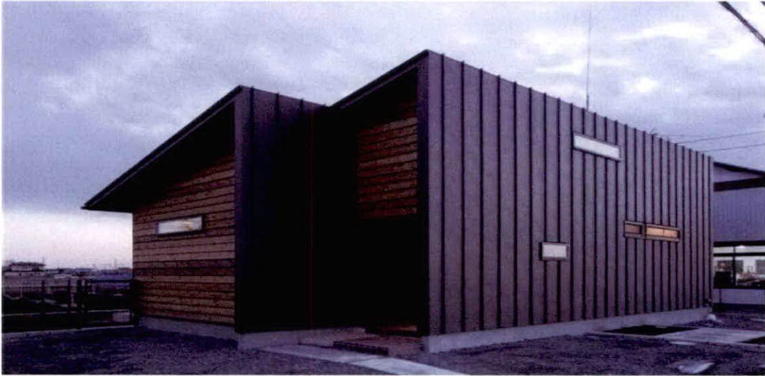
This is an example of zinc standing seam and cladding. It's a random illustration of how these materials appear in combination.
